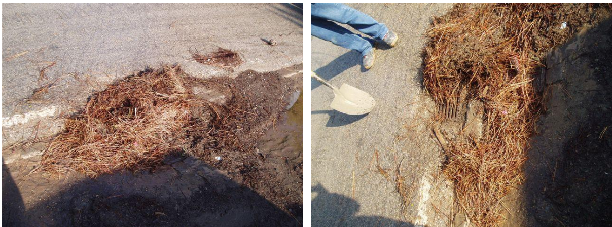
Figure 2.6 Sewer sink clogged due to accumulation of leaves and pine tree needles carried by storm runoff (Quinta do Lago, Loulé, Portugal). The sewer sink trash rack was found completely covered after a flooding event which occurred on the 29 th September 2008 (left). A worker removes the accumulated leaves and pine tree needles, uncovering the sewer sink trash rack (right).
