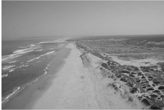
Figure 4.1 - View from the air with Leirosa at the top, pressure chamber of the emissary in the middle and the part of the dune in front of the pressure chamber that was partly repaired in January 2006 (Antunes do Carmo).
