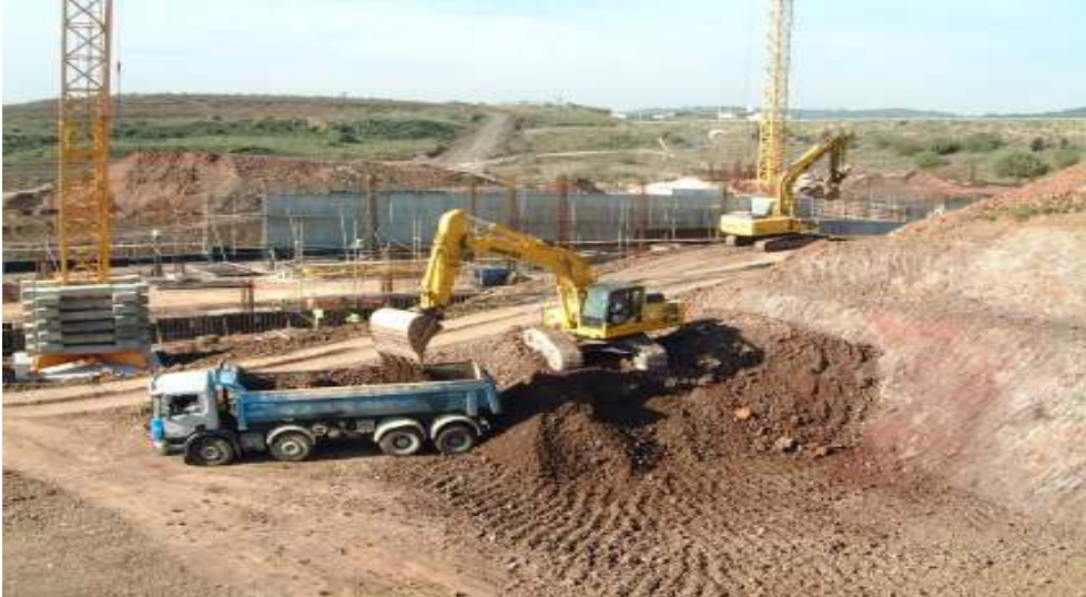
TERRAPLENAGENS GERAIS DOS LOTES 1, 2, 3 e 4 LOURES BUSINESS PARK
