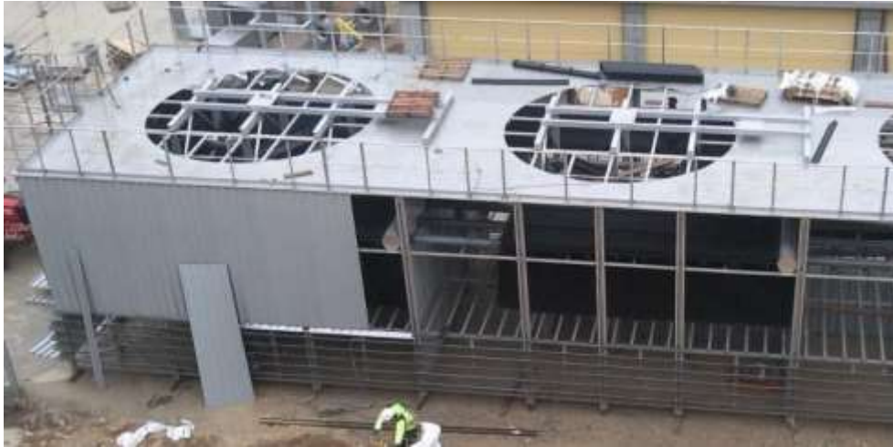
Fig. 1: Cooling tower construction.
