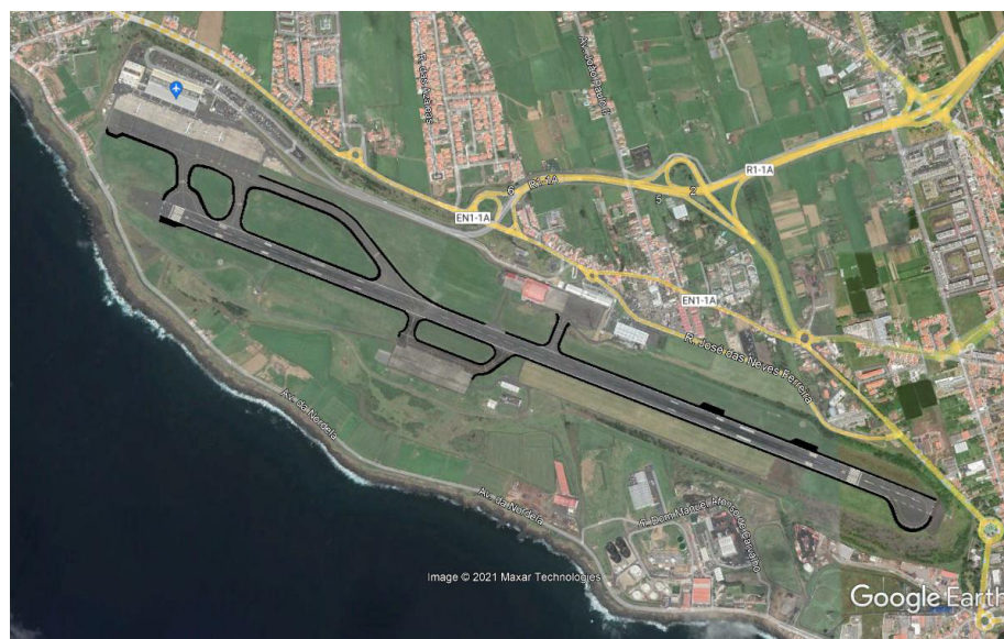
Figure 2. Installation aerial view overlaid with implementation zone.
