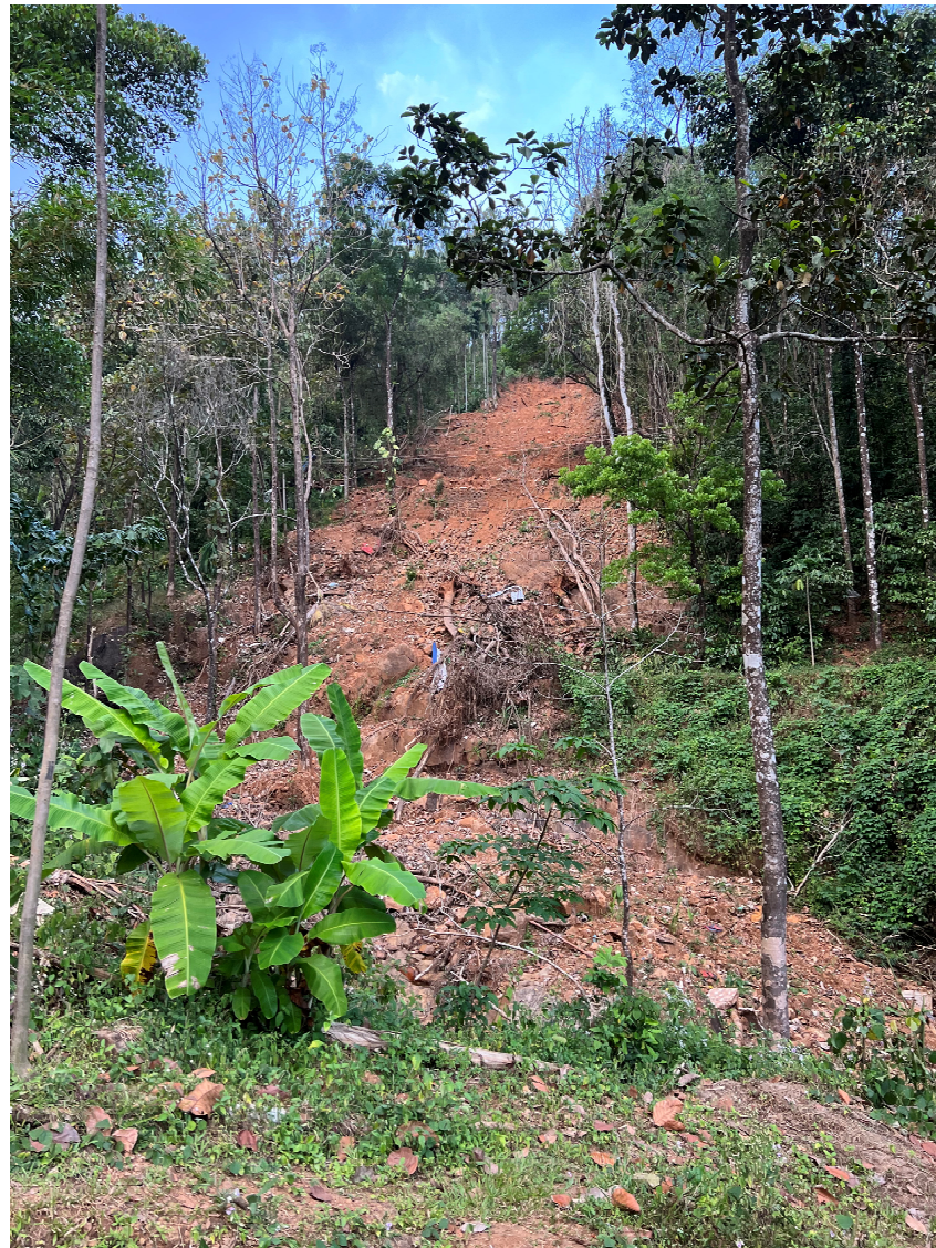
Figure 1. The Kavali landslide resulted in the demolition of one house and the death of six people.
