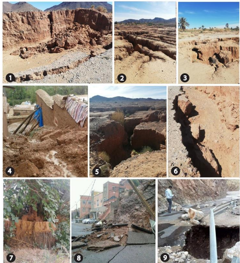
Figure 9. Photographs showing the severity of water erosion and associated floods in the study area: (1) Taghia, (2) Taghzout, (3) Ait Iala, (4) Ait Hani, (5) Tilouine, (6) Taghia, (7) Asfalou, and (8,9) Tizgui.
