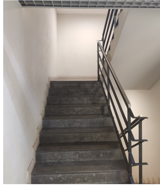
(b) Featureless staircase.
