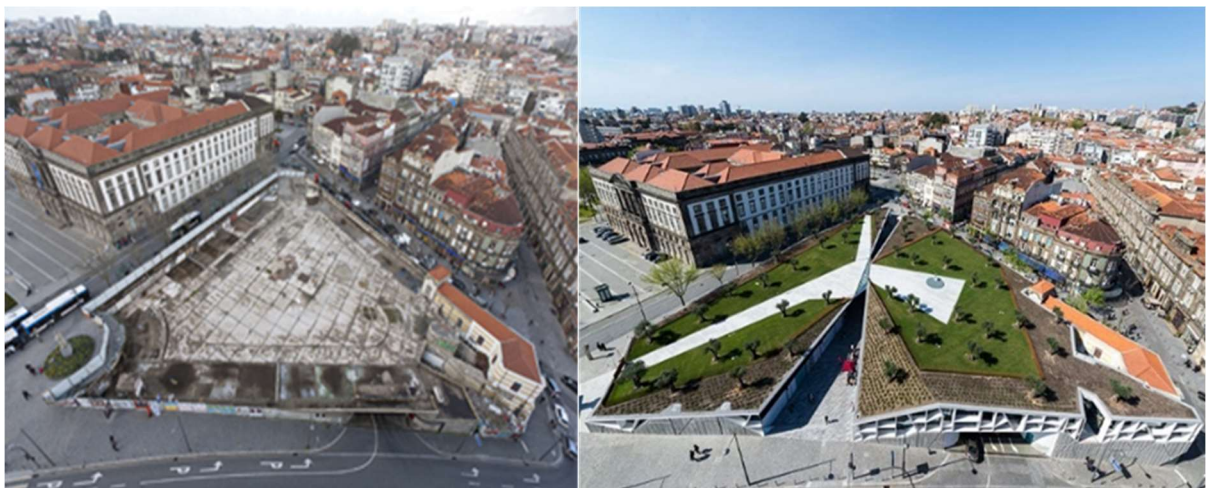
Figure 2.5 - Praça de Lisboa in Porto - construction stage (left) and green roof (right) (Source: JPN and SustentArqui)
