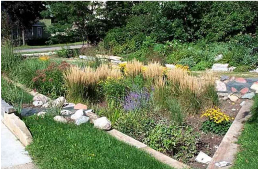
Figure 2.8 - Rain Garden (Source: NWRM)
