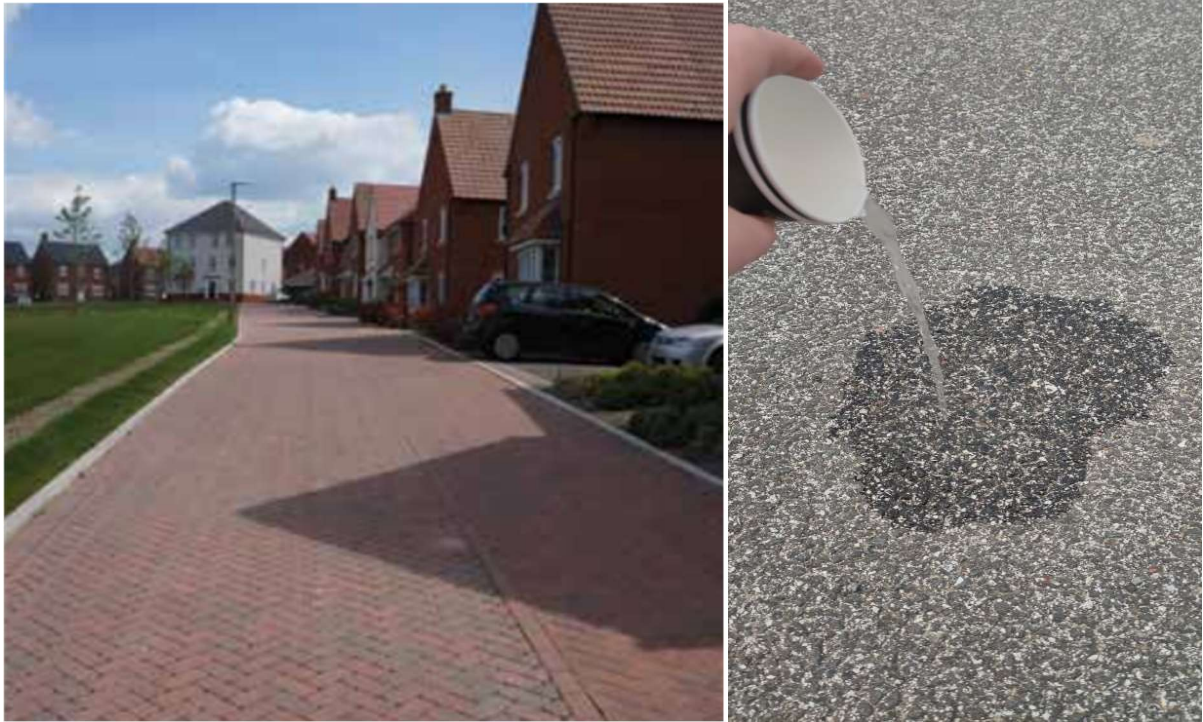
Figure 2.6 - Types of permeable pavements (Source: SUDS manual and author)
