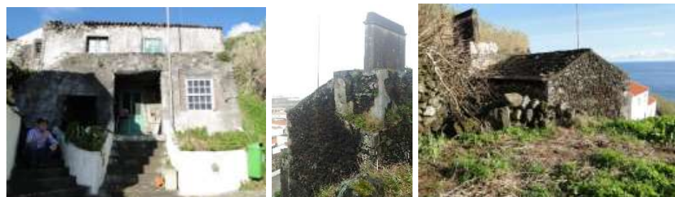
Figure 16. General views of the building surveyed.
