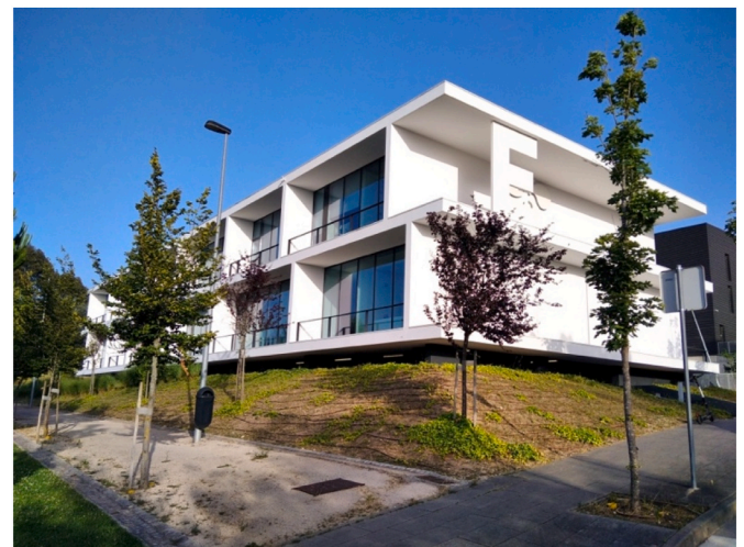
Fig. 3. IPN's 'TecBIS building E' in Coimbra, Portugal.
