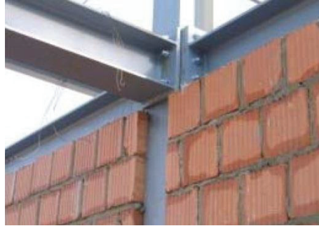
Figure 7.30: Masonry infill panel execution detail (Markulak et al. , 2008)
