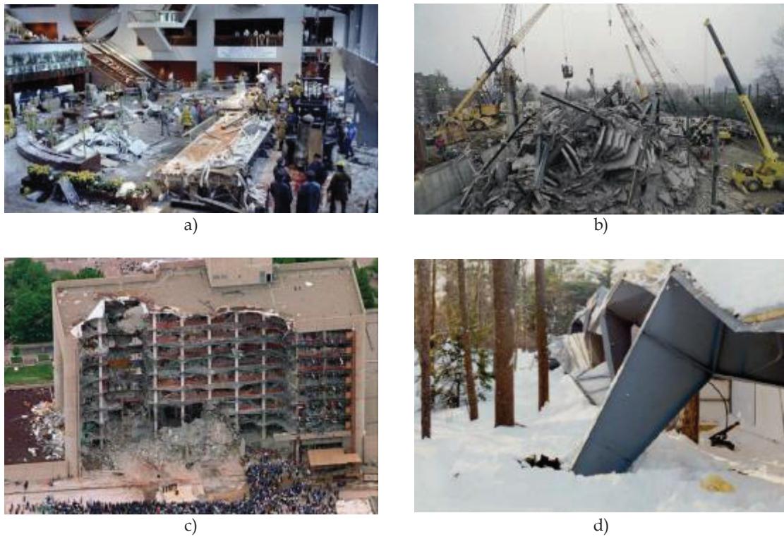
Figure 1.3: Case studies of progressive collapse (National Institute of Standards and Technology, 2007): a) Kansas City Hyatt Regency Hotel; b) L'Amiance Plaza; c) Alfred P. Murrah Federal Building; d) Jackson Landing Skating Rink
