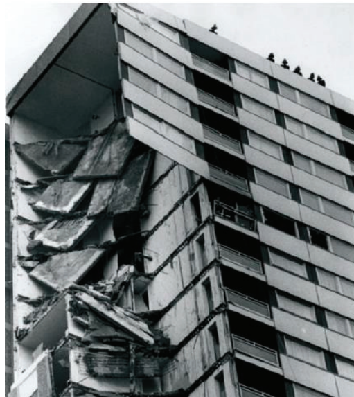
Figure 2.4: Partial collapse of the Ronan Point tower
