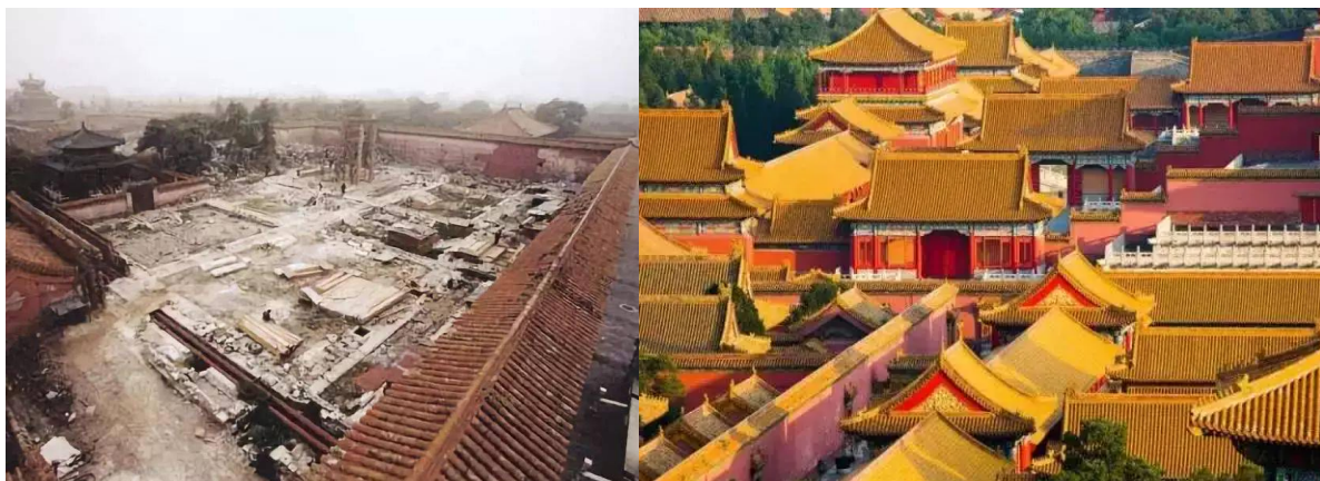
Figure 19 – The natural deterioration of the Forbidden City
