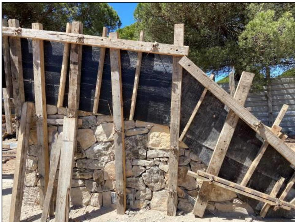
Figura 5.10 – Amostra pronta a betonar.
