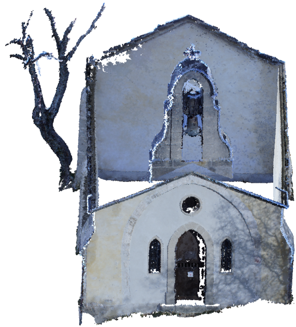
(g) House without Roof.
