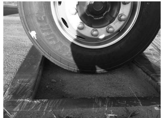
Fig. 10 – Interaction between tire and pothole.
