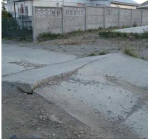
Figure 2.5: Uprising of the pavement in El Ovejero, Punta Arenas (adapted from Vasquez, 2012)
