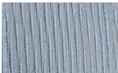
Figure A.10: First layer of reinforced base coat.
